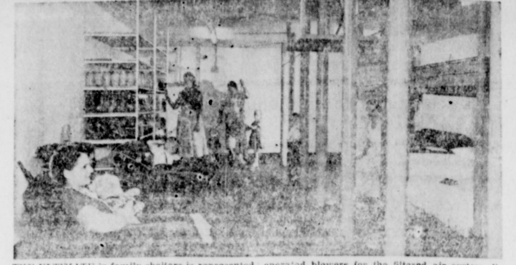
THE ULTIMATE in family shelters is represented by this large and luxurious unit built by steel contractor Earl W. Reichert of Baile Creek, Michigan. The $10,000 structure has a 50-foot well, private electric generating plant, electric and hand-operated blowers for the filtered air system. Its steel reinforcement prepares it for use as a blast as well as fallout shelter. However, a small family fallout shelter may be built for a fraction of what this shelter cost. (Baile Creek Enquirer and News Photos)
