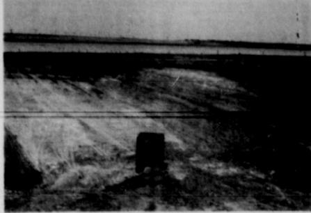
SCREEN. . . In the middle of the picture can be seen the trash screen guard on a suction line. This tailwater pit is being constructed by Sam Rundell on the playa lake near Missouri Beef Packers' plant, Friona.
