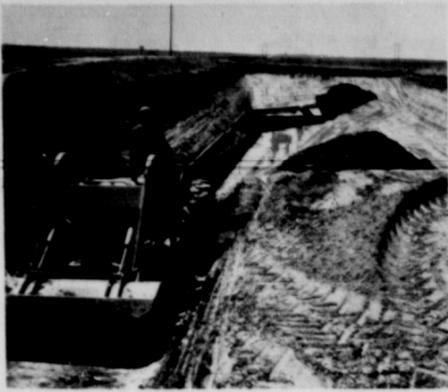
PIT CONSTRUCTION. . . A backhoe is shown digging a trench for a pipe for the tailwater pump on the L.L. Norton farm four miles northeast of Farwell.
