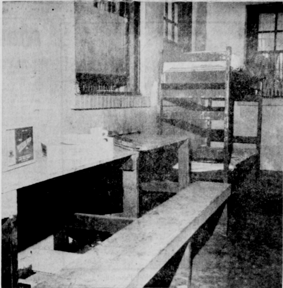
Interior view of jail.
