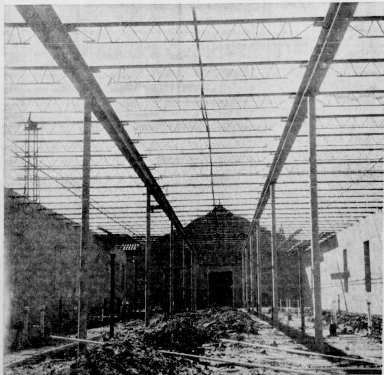
Roof beams in place . . .
