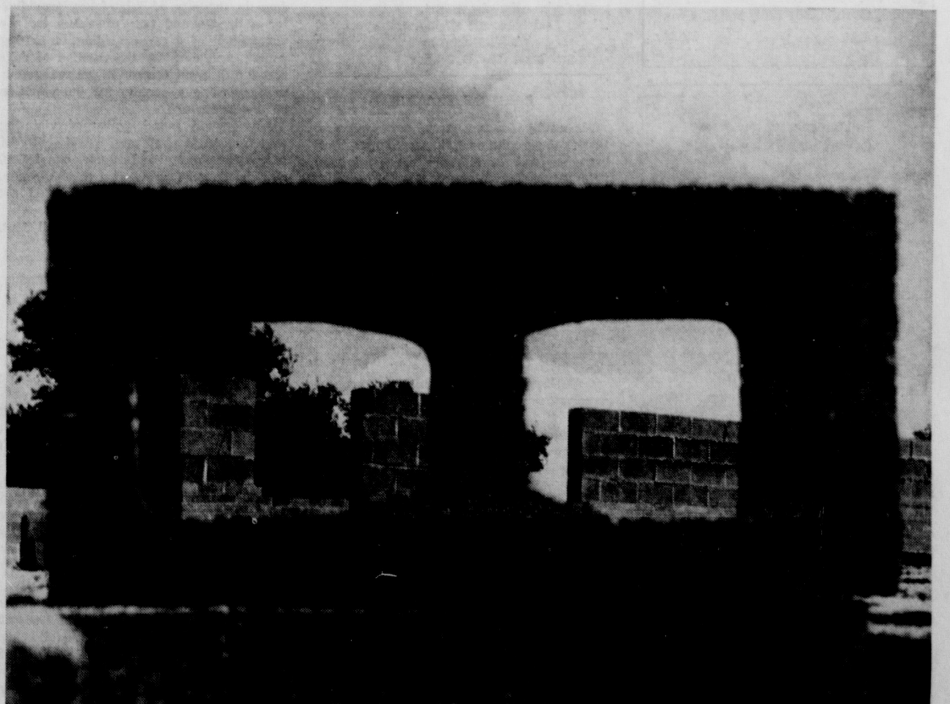
Post office work continues . . .
