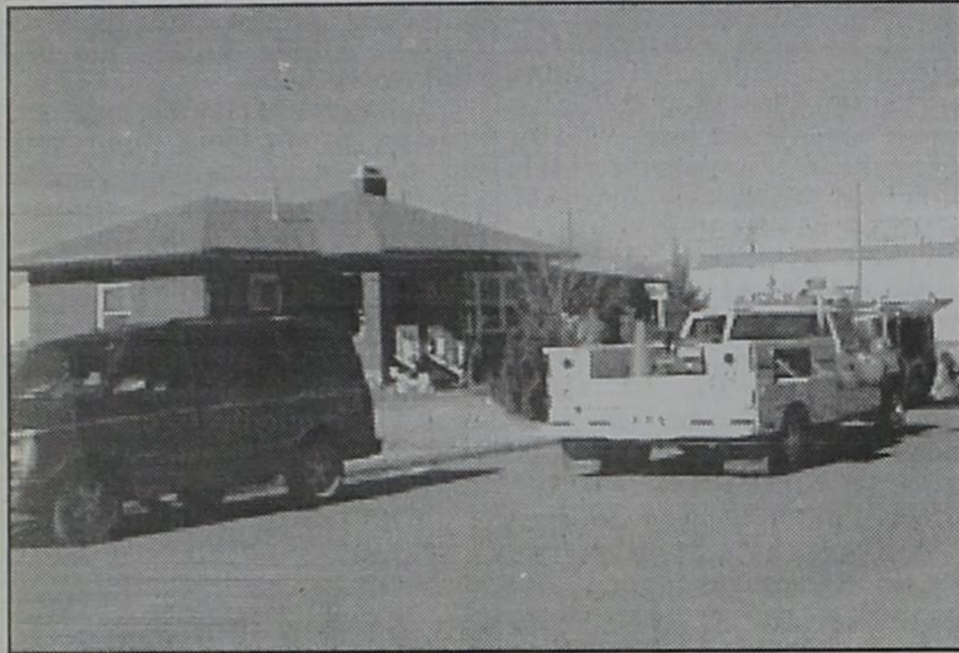
THE FRIONA FIRE DEPT. was called out on New Year's for a fire at 913 Washington Street. A fire in the house's attic was probably of electrical origin. The house was Friona's first brick home.
