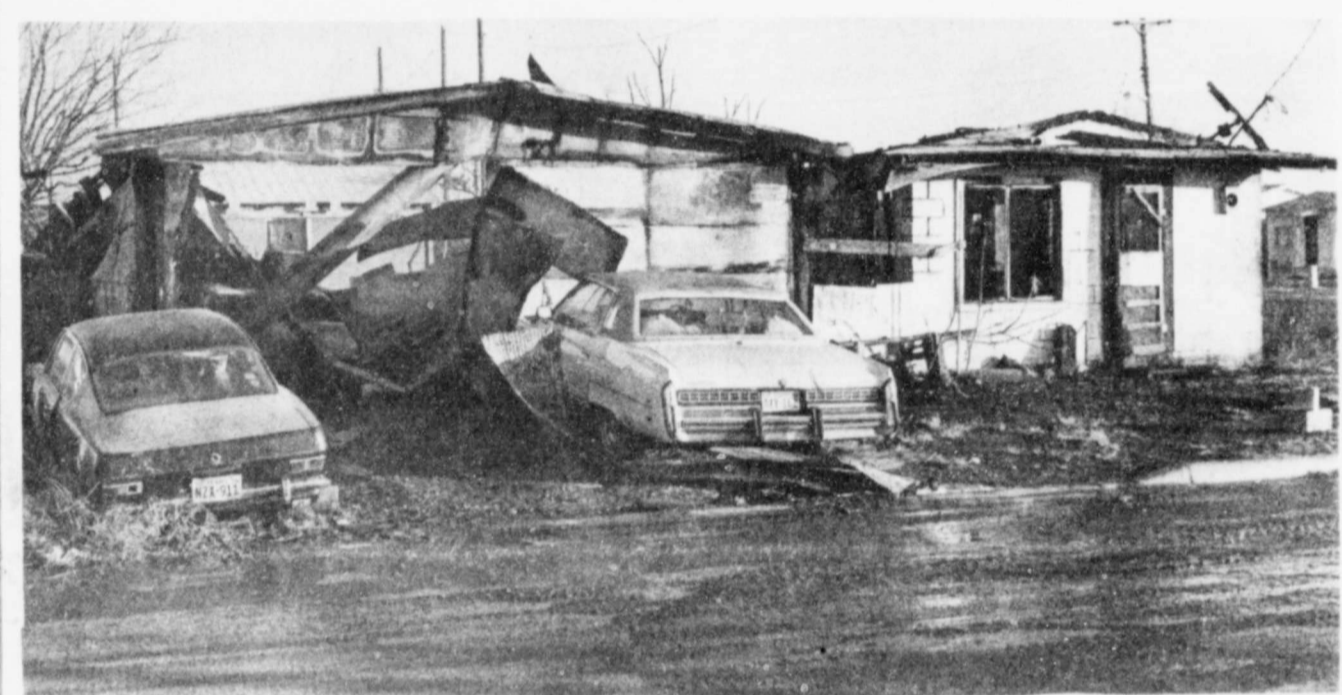
THE REMAINS of a garage fire that broke out early Tuesday morning. The entire structure was gutted and the two cars inside were totally destroyed. Floydada Firefighters responded to the fire 4:30 a.m. It took about 20 minutes to get the fire under control and about another hour to completely extinguish the blaze. Cause of the fire is not known, but it is believed to have been caused by a wood stove. The fire will not be investigated for arson.
