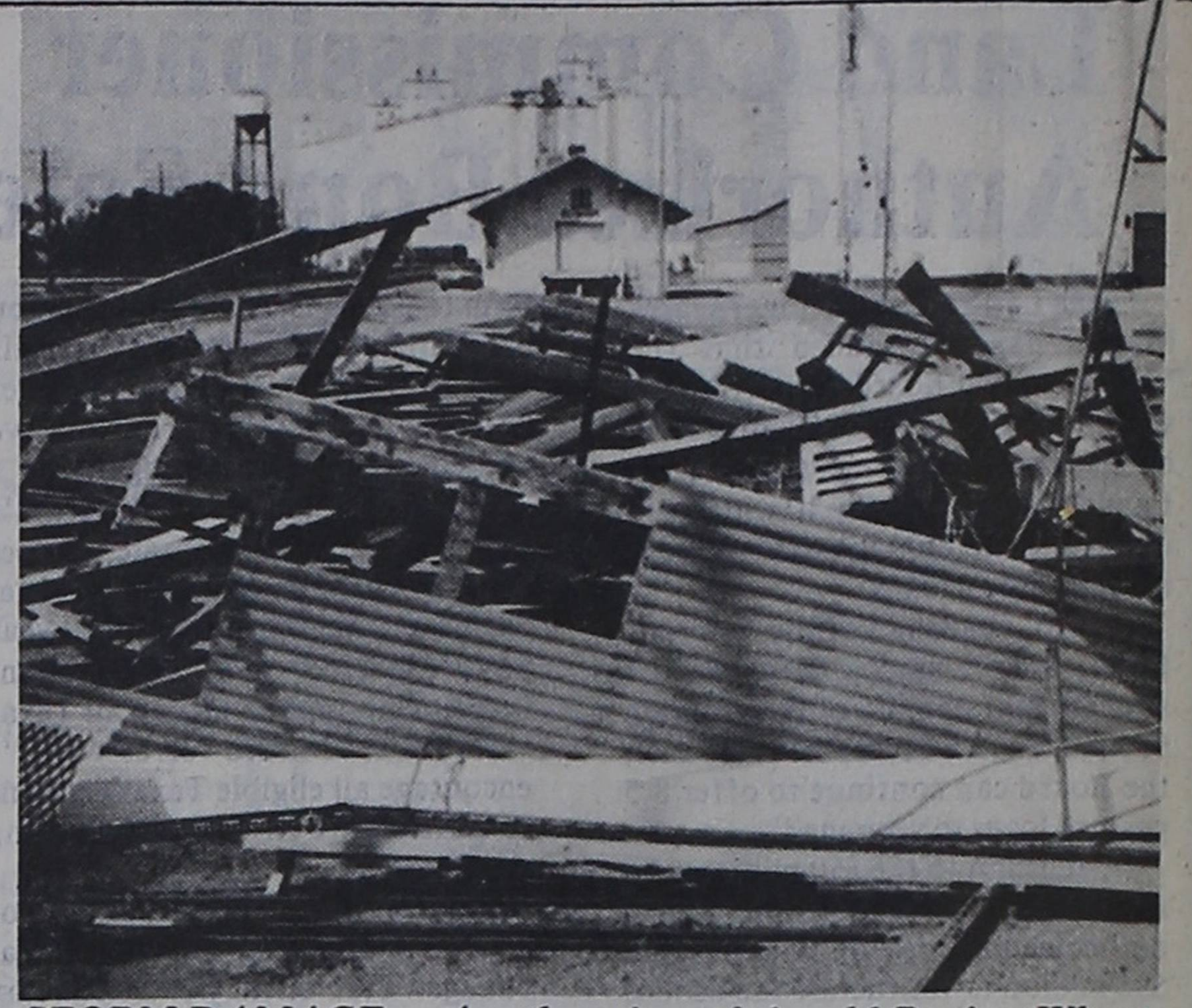
STORM DAMAGE....Another view of the old Bovina Wheat Growers warehouse, demolished by an apparent twister Tuesday evening, shows the wreckage that was left. Nearby buildings were spared, as the empty building was the storm's main target.
