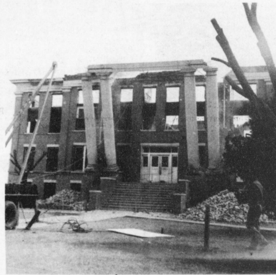
DESTROYED -- In March 1949, the Floyd County Courthouse, built in 1912 of pressed brick with reinforced concrete floors and stairways with marble treads, was burned beyond repair as contractors worked to replace a metal dome topped by four clock faces and reroof the building. Temporary quarters were set up in the Ag building and a hurriedly constructed frame structure until rebuilding was complete in March 1951.
