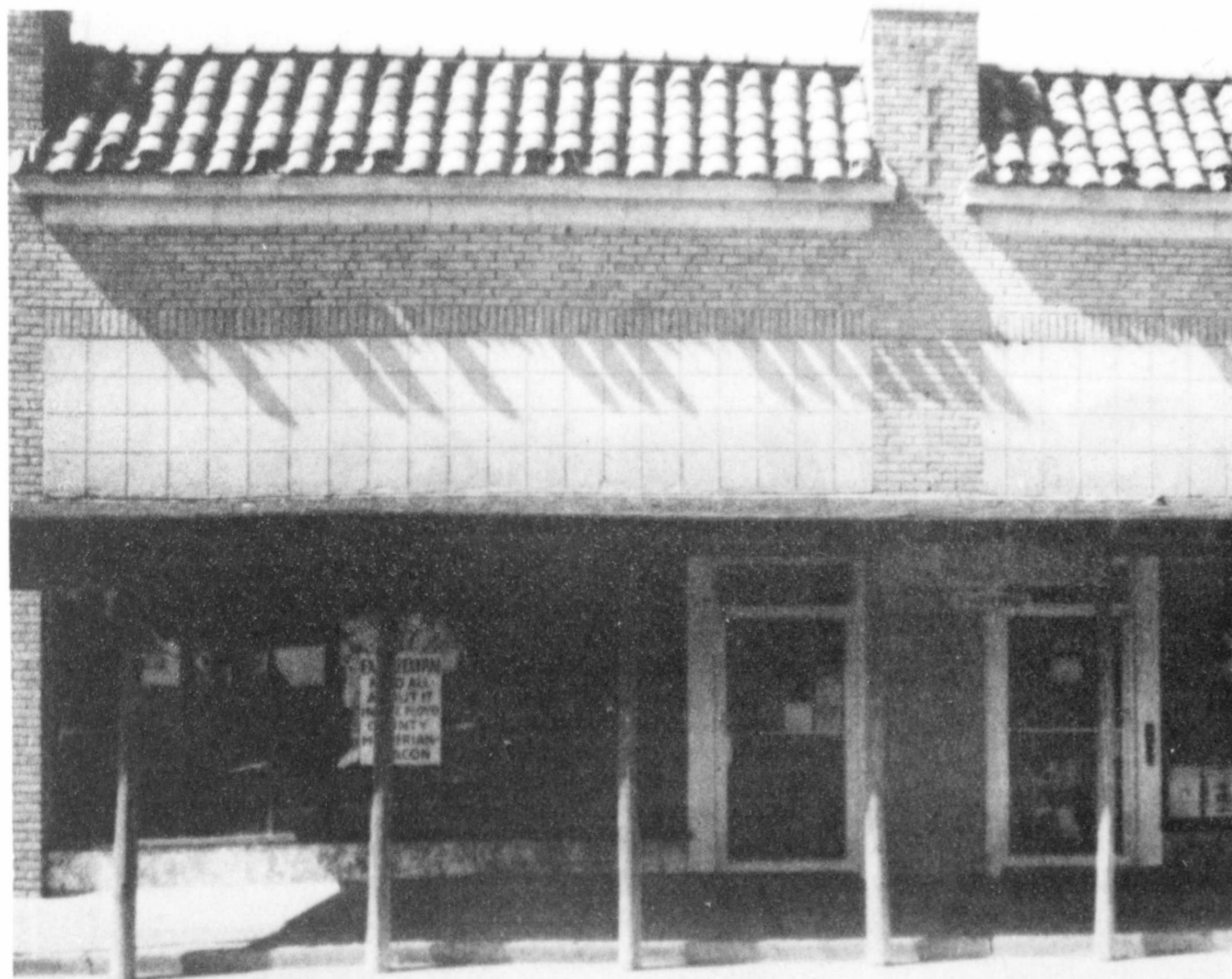
CURRENT BUILDING HOUSING THE FLOYD COUNTY HESPERIAN-BEACON AT 111 E. MISSOURI.
