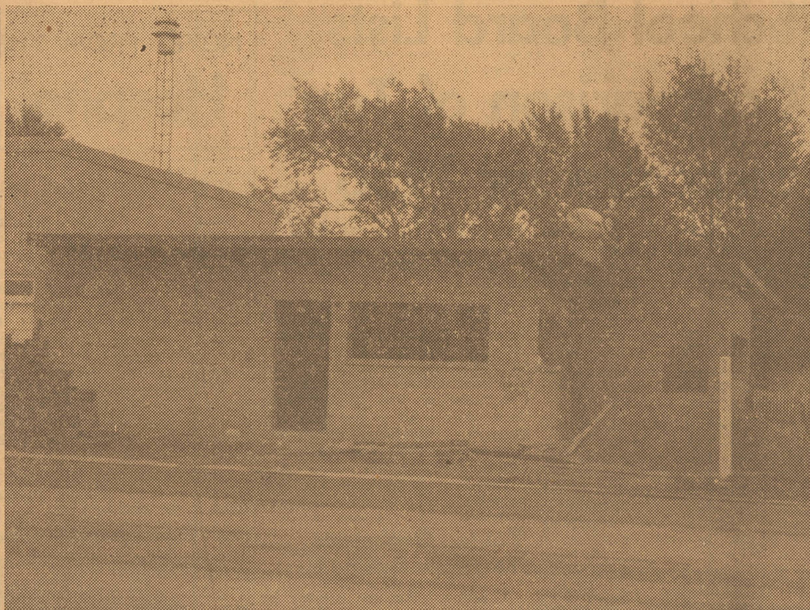
MOVING ALONG—City officials expect to be moving into this modern new building by the middle of next month if everything progresses satisfactorily. The new city hall adjoins the fire station and is being built at a cost of over $40,000.
