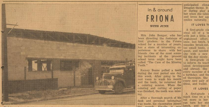
Taking shape is the new building of Jones Motor Company on Highway 60 in eastern Friona. The building, which is being built of tile and brick on a steel and concrete framework, is next to the present Jones Motor Company building.
