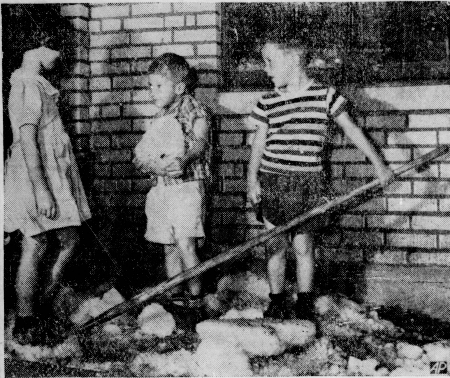
These youngsters at the Hendrick Home for Children at Abilene, Texas, tried their hand at constructing an ice man of hailstones piles in the corner of the building. The window behind them contains several of the 800 window panes that were broken by the storm. Left to right are: Bobby Jean McKinney, 6; Dale Hooks, 6; and Don Sedberry, 4. (AP Photo).
