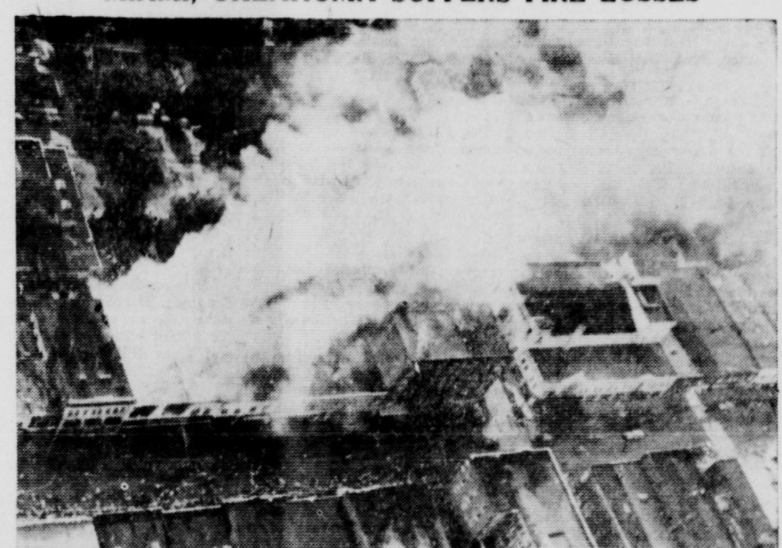
Smoke columns up as fire departments from other Oklahoma, Missouri and Kansas cities fight a fire which threatened the business district of Miami, Oklahoma. The fire, believed to have originated in a ventilating fan of a paint store, spread rapidly and endangered the entire block before being brought under control. The estimated damage was $750,000. (NEA Telephoto).
