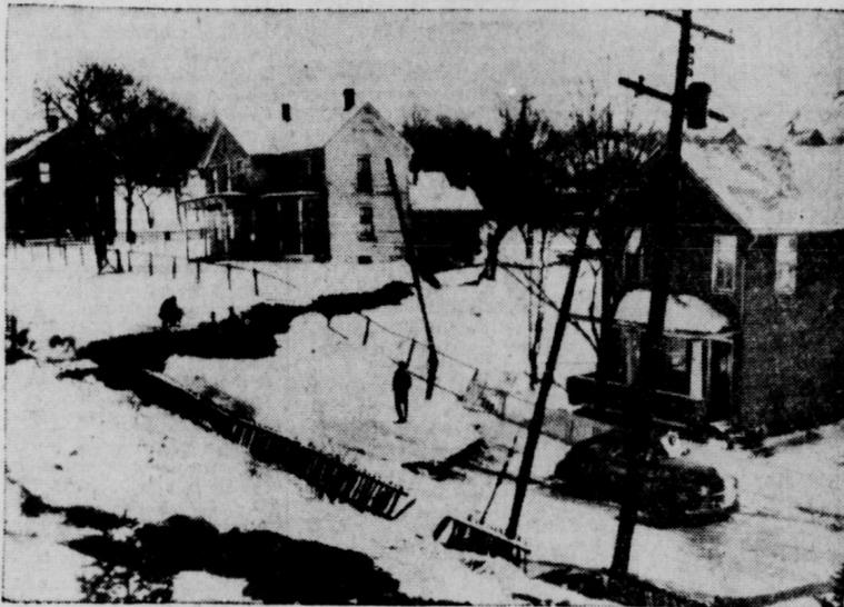
Kane Street in Carbondale, 20 feet after the collapse of an underground anthracite mine shaft. Four persons were injured and 14 homes were damaged by the collapse. A warning rumble preceded the cave-in, waking residents and enabling them to escape. — ACME.
