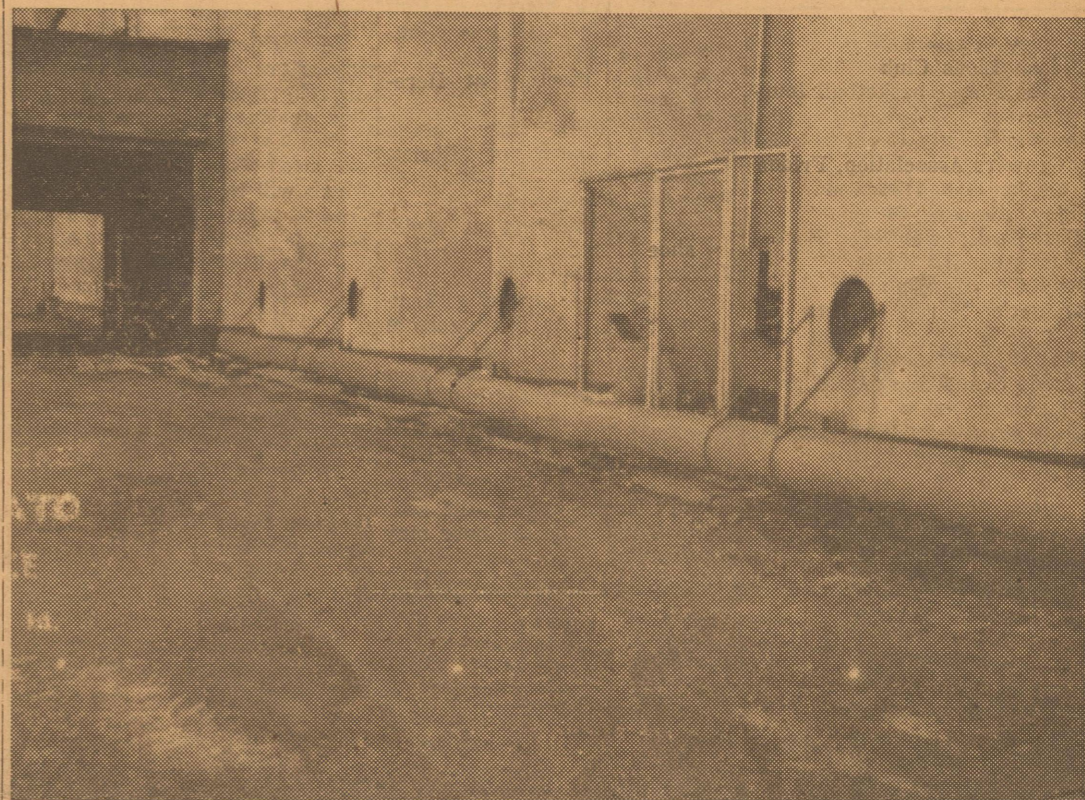
NEW GRAIN DRYER—Friona Wheat Growers Elevator has started using the new grain dryer pictured here. Work is still going on finishing the shed for the dryer. The machine is automatically fed and has automatic controls for temperature.
