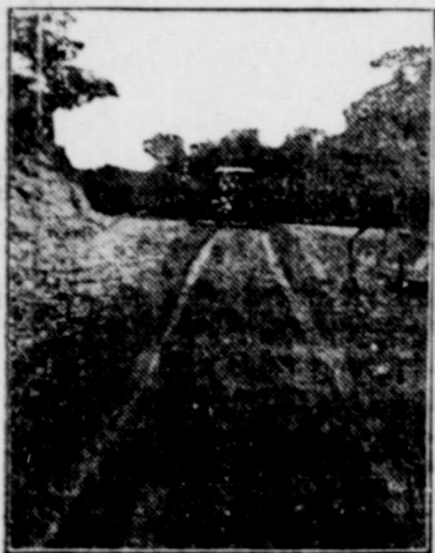
A Sandy Road After Grading Before Improvement With Crushed Stone in Town of Delton, Sauk County, Missouri.
