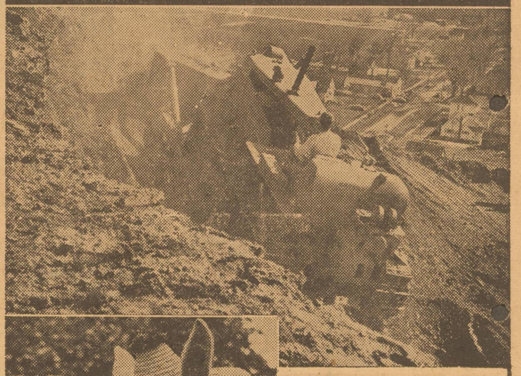
GOUGING Foothold on side of mine waste pile above Wenona, Ill., D8 prepares site for emergency warning radar station. (CNS PHOTO)
