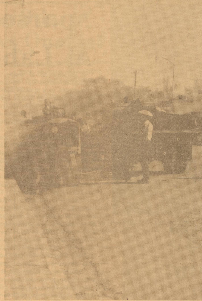
DUSTY DUSTY WORK --Clyde Fields, hidden amidst the dust on top of the street sweeper, guides the machine down the curb along Main Street in Friona Tuesday morning in preparation for retopping the curb area of the Street.
