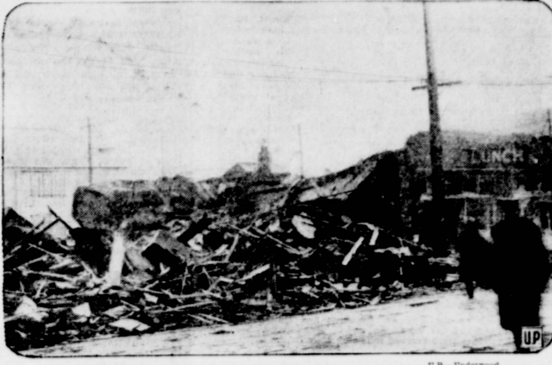
The ruins of a furniture and music store in Detroit where an explosion wrecked an entire city block, injuring several and doing damage estimated at over $500,000.
