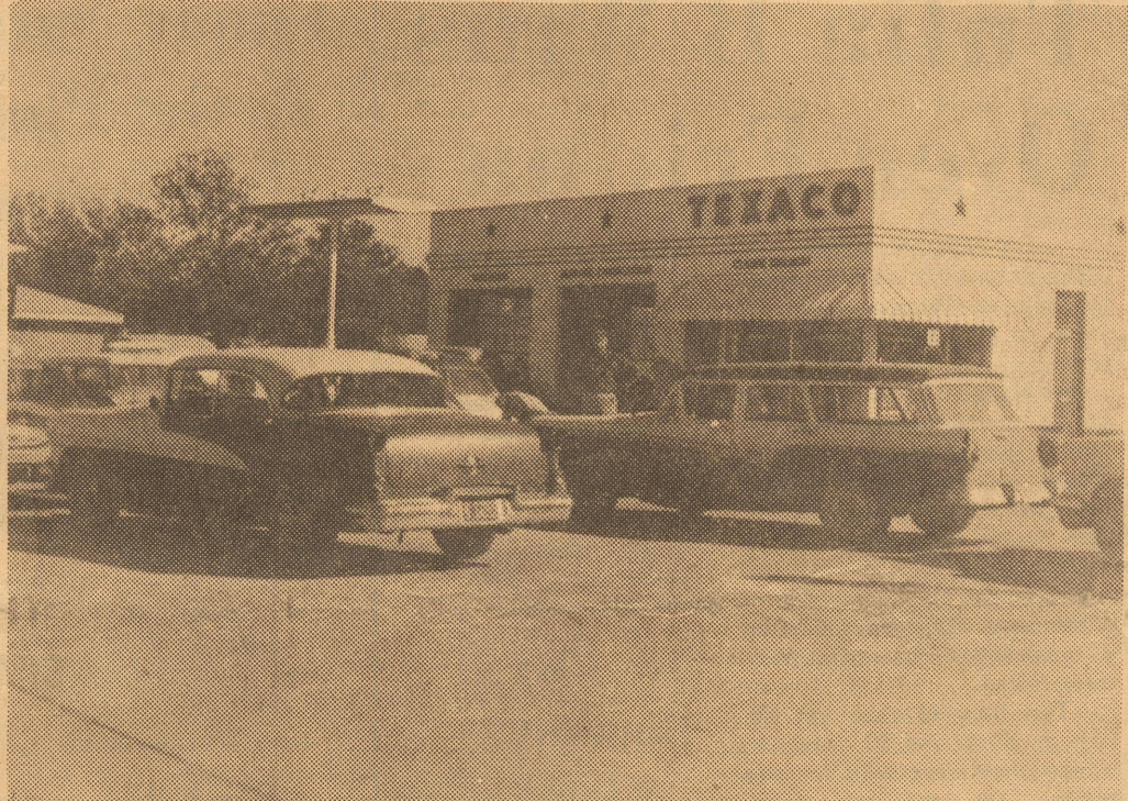
SENIORS GOT SNOWED UNDER--Saturday was a busy day at Edelson's Texaco Station when the Seniors of Friona High took over the station for a one-day stand. This scene was typical of the crowd which swamped the station all day long.
