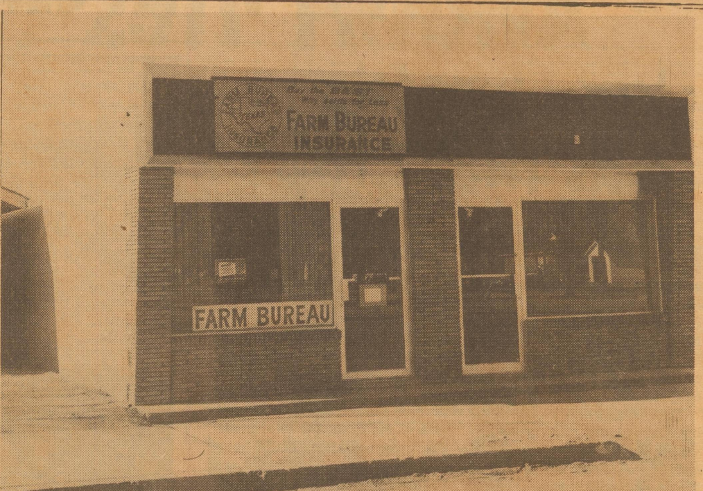
NEW HOME of the Parmer County Farm Bureau is this attractive office building in Friona. It was occupied by the organization and Service Agent Raymond Euler two weeks ago. Bill Garrett, Farwell, is contractor.
