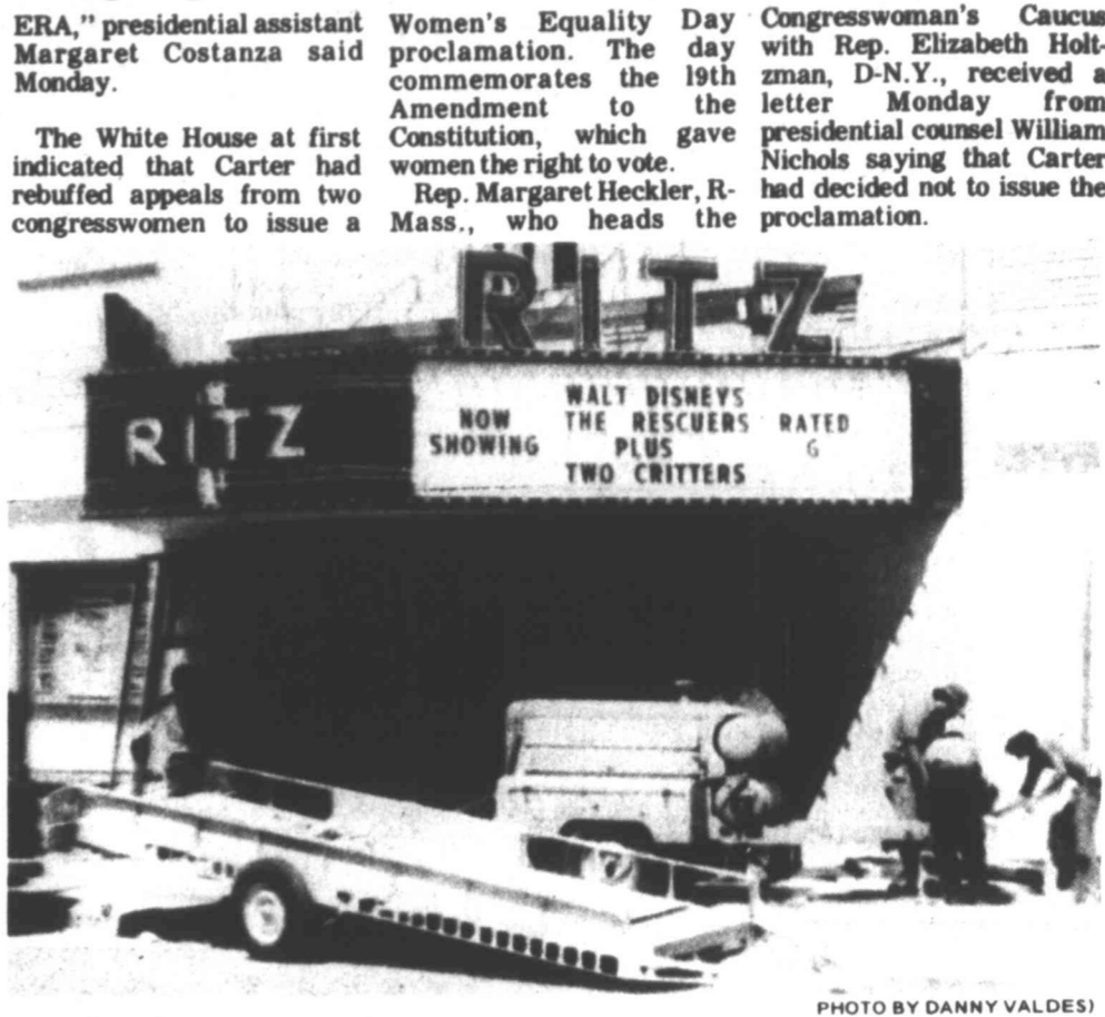
BUSINESS AS USUAL TODAY — For the first time in many years, the Ritz Theatre was closed to the public Monday. Workers raced to complete work on the entrance to the historic old theater. The movie house reopens today with the film featured on the marquee here. Owner Ike Robb said the present plans are to open the Ritz's unique dual screen concept Friday, Sept. 2, at which time he hopes to feature top-rated movies on both screens. The main section of the theater seats 468 while there are 241 seats available in the balcony. Moviegoers will buy specially-colored tickets to see either of the two attractions booked by management.
