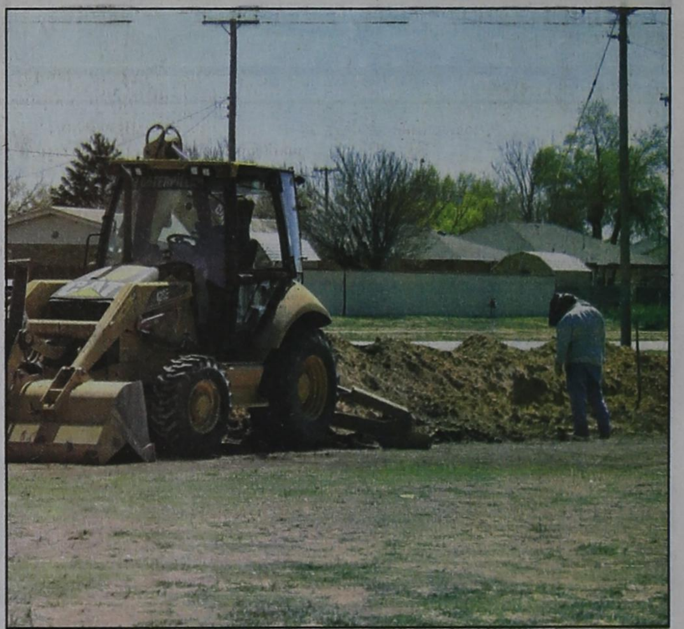
City employee Salvador Garcia used the ditcher to dig a trench to install the sewer line at Reeve Lake for adding another 10 spaces in the city RV Park. The work should be complete by next week he said. The city anticipates the 20 RV spaces will be full for much of the year by wind turbine project workers.
