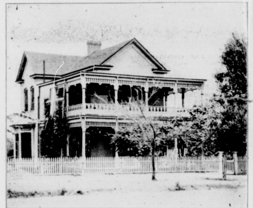
RESIDENCE OF J. R. HAMILTON, SAN ANGELO.
