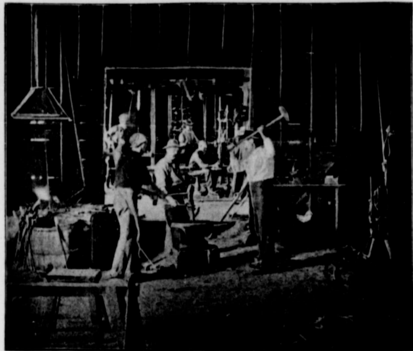
INTERIOR OF COPELAND & CO'S MACHINE AND BLACKSMITH SHOP
