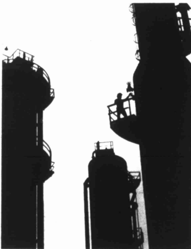
LOFTY PERCH — Amid the tall towers at Tenneco Inc.'s Petro-Tex chemical plant in Houston, Assistant Stillman Tommy Drouillard appears small indeed as he operates a valve from this lofty perch. Petro-Tex is a leading producer of MTBE, a blending agent that increases the octane rating of unleaded gasoline.
