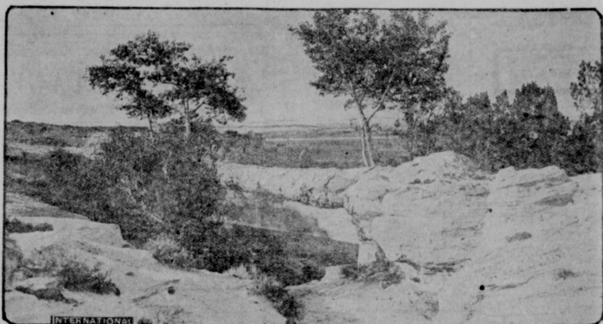
So many persons wanted to enjoy the thrill of creeping across this natural bridge near Tucson, Ariz., that the bridge, which is a petrified tree, showed signs of weakening. Engineers were called on and reinforced the bridge with concrete.
