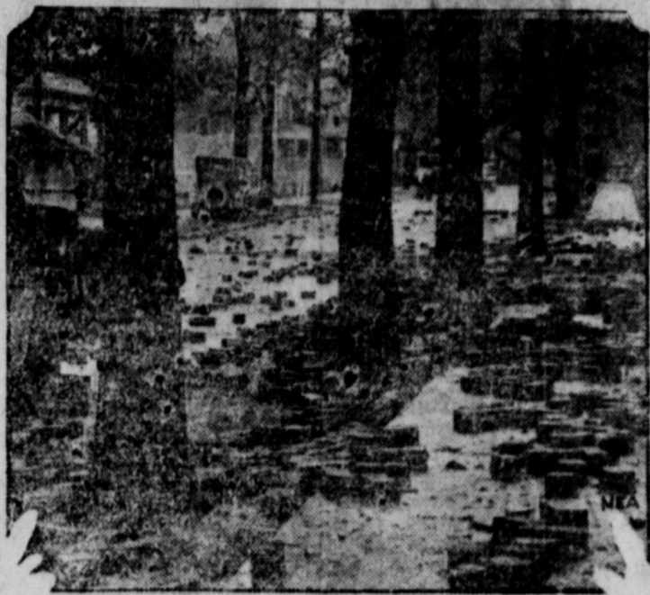
They had a heavy rain in Detroit—almost a cloudburst—and it flooded dozens of streets. Streets that were paved with wood or composition blocks suffered heavily as the blocks floated away and were scattered all over the city when the waters subsided.
