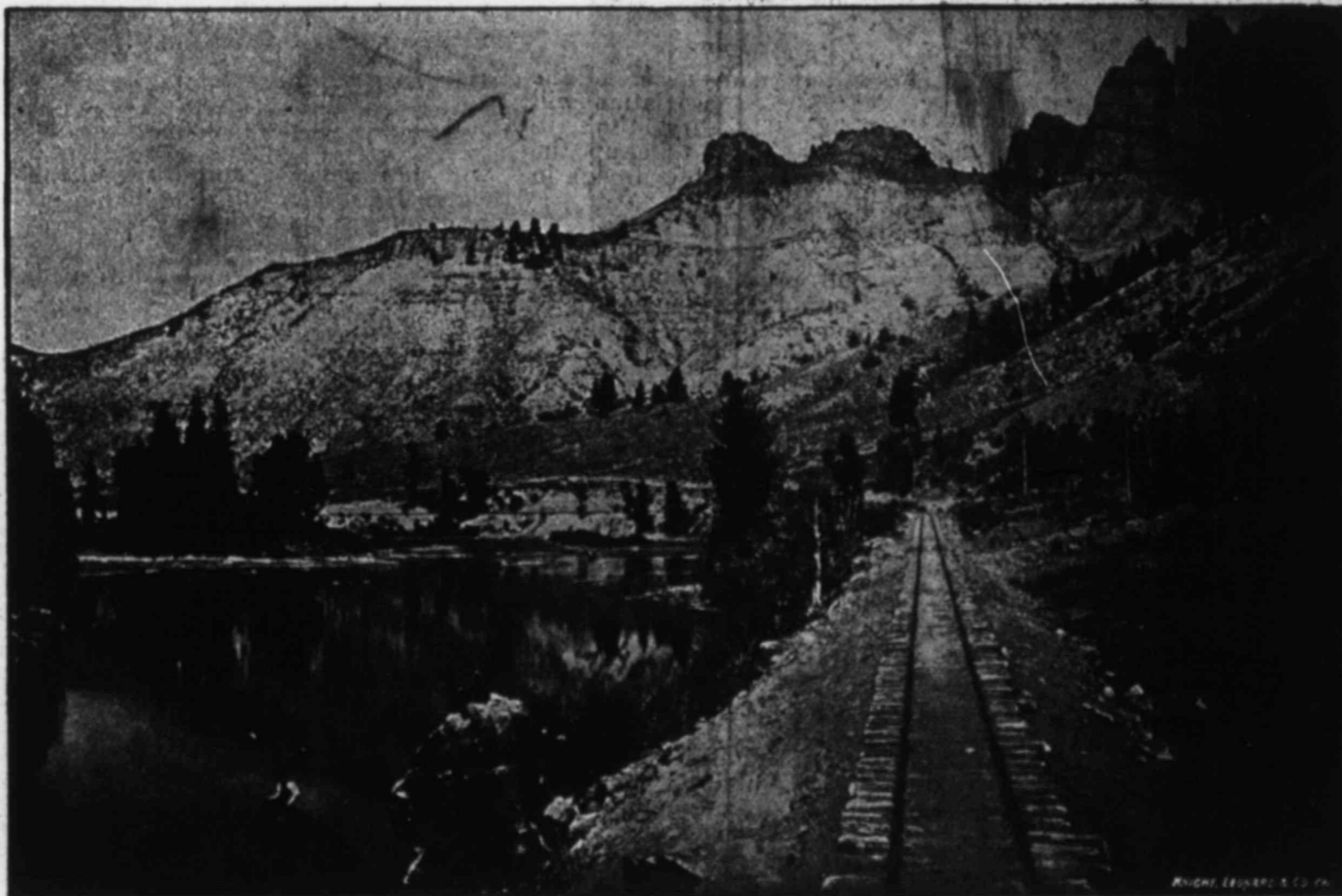
APPROACH TO BLACK CANYON, COLORADO Courtesy Denver and Rio Grande Railway
