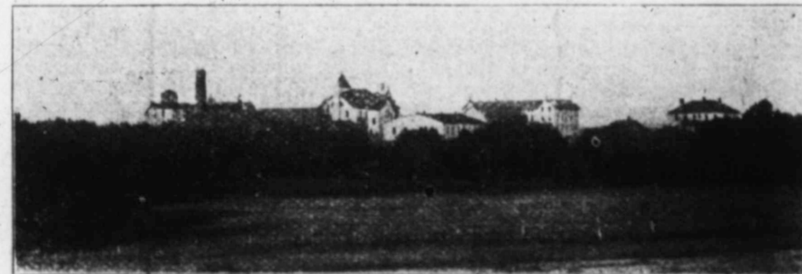
Looking North, Showing Windmill and Tank.
