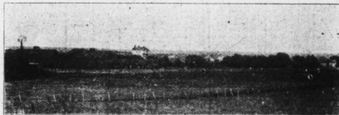
View of Main Buildings Looking Northeast.
