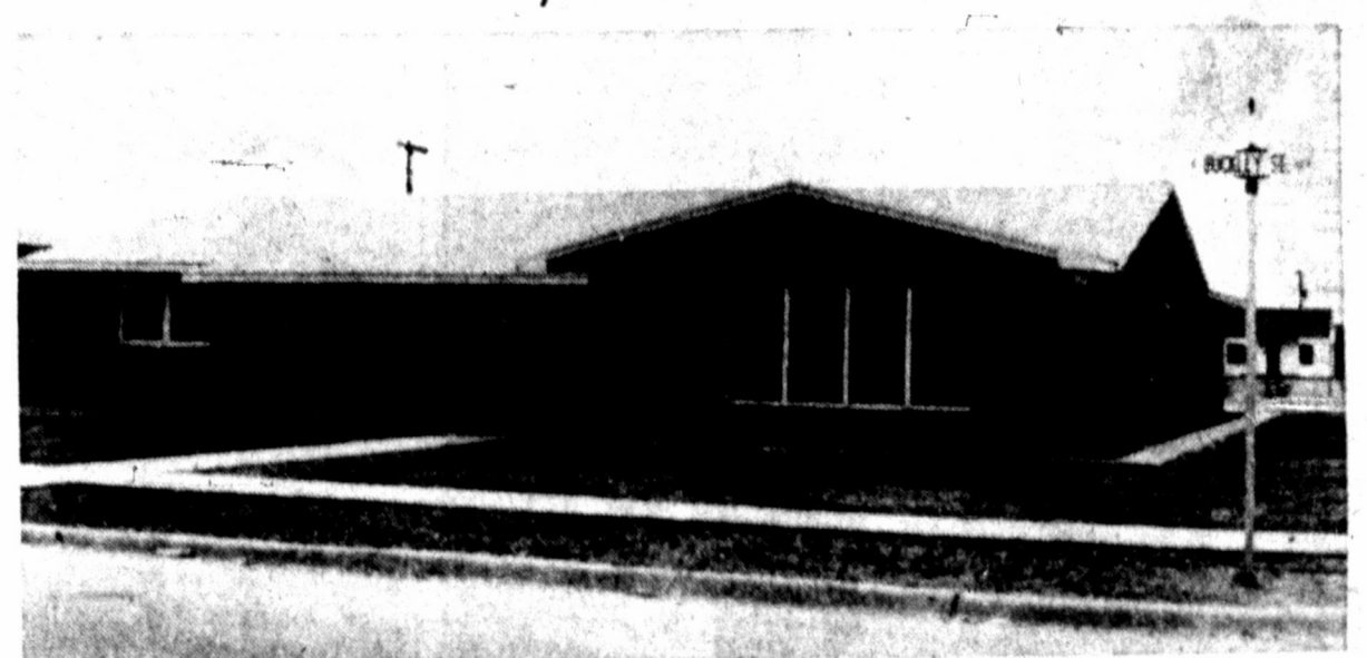
ROMAN BRICK BEAUTY — This is the new home of Mr. and Mrs. P. R. Cates at 902 E. Buckley. Constructed of Roman brick with white slate roof, this home has many unique features within its 3900 square footage. One of these features is the lack of west exposure — only one small window faces onto the west. Notice the protected entry way and the neat brick planter at the front of the house.
