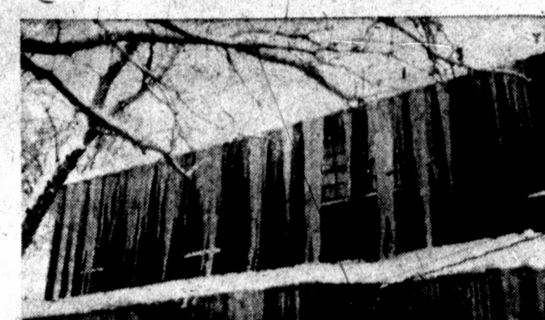
STALACTITES? Yes, but of solid ice? These giant icicles formed on the roofs of the two story home of Mrs. Tom May, 202 E. Carwell. Icicles from the top story hung to the roof of the ground story, and icicles on the roof of the ground story touched the ground, some eight feet in distance. Mrs. May said the huge formations were probably caused from heat from three heating units in her home. Many people stopped Saturday and Sunday to inspect the icicles.
