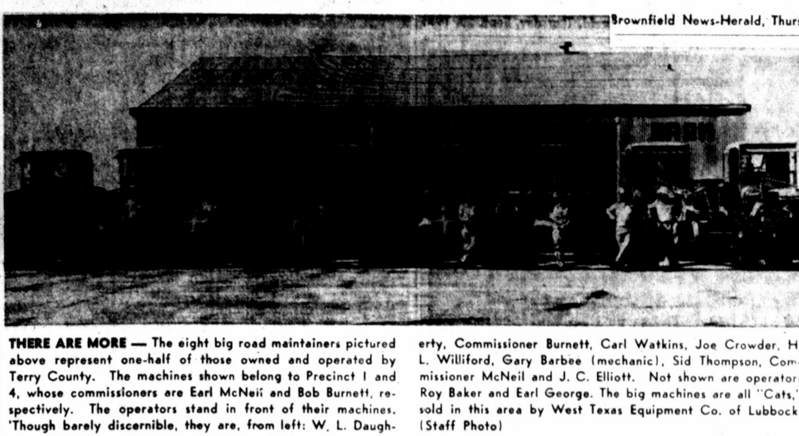
THERE ARE MORE — The eight big road maintainers pictured above represent one-half of those owned and operated by Terry County. The machines shown belong to Precinct 1 and 4, whose commissioners are Earl McNeil and Bob Burnett, respectively. The operators stand in front of their machines. 'Though barely discernible, they are, from left: W. L. Daugh-
