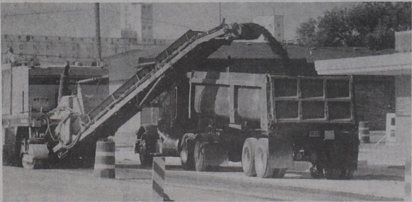
CHEWING UP THE PAVEMENT.....TX/DOT contractors chewed up the asphalt on the west side of Main Street last week in preparation for repaving. Rain halted the construction for a couple of days, but the progress seems to be moving along at a good pace. (Ron Carr Photo)
