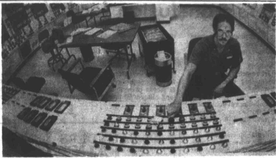
OUT OF CONTROL ROOM — A technician sits in the multi-million dollar control room of a nuclear fuel reprocessing plant in South Carolina that's being forced to shut down this summer because of no business.
