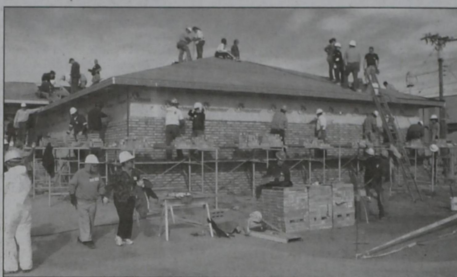
Bricklayers and roofers at work Friday
