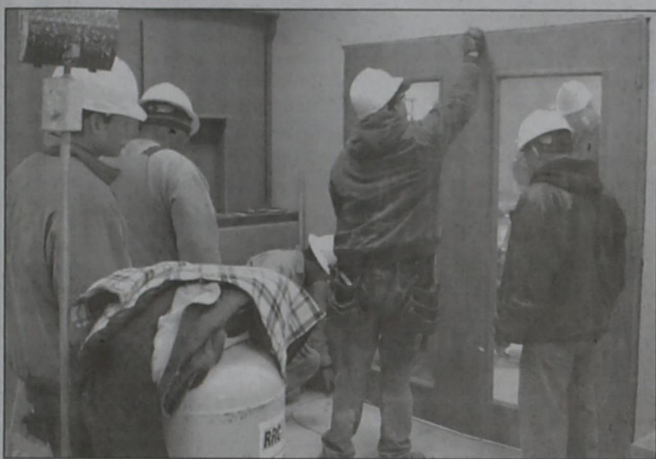
Workmen hang doors inside.
