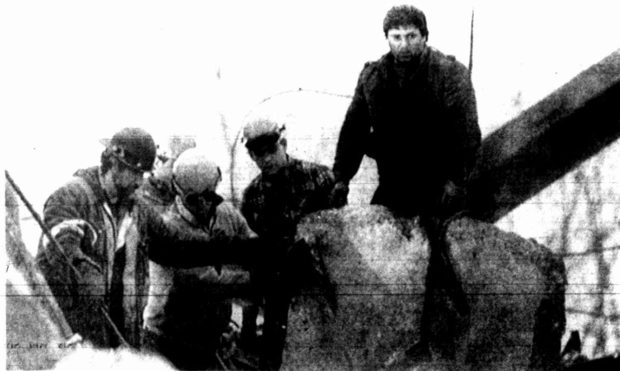
Rescue workers prepare to move a chunk of concrete as the search continued for missing construction workers in the wreckage of an apartment building that collapsed Thursday in Bridgeport, Conn. Nine were known dead and 19 were missing in the collapse.
