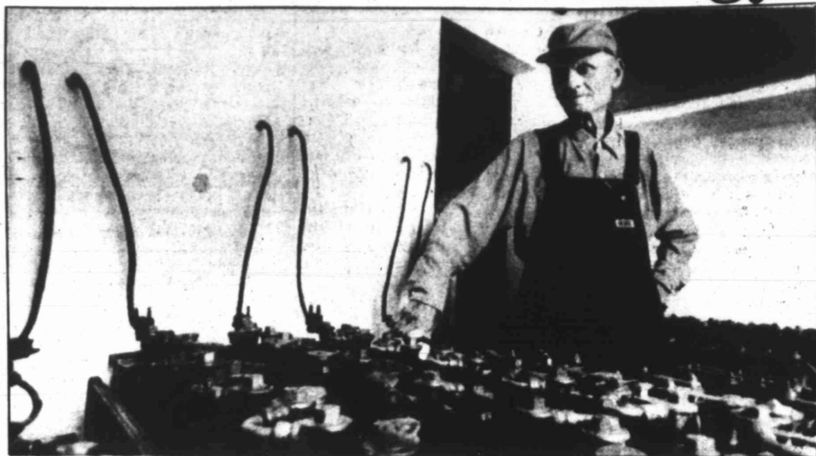
WOODWARD, Iowa — John Lorenzen, who has run his central Iowa farm on power from wind chargers since before the Depression, checks connections on the dozens of huge batteries that store power for times of low wind. Lorenzen, 81,
