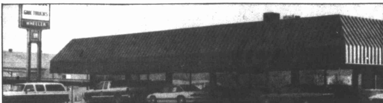
Wheeler Motor Company, now in a newly remodeled building, has been at the same location since 1948. The Wheelers stressed that the number one goal of this third generation business has
