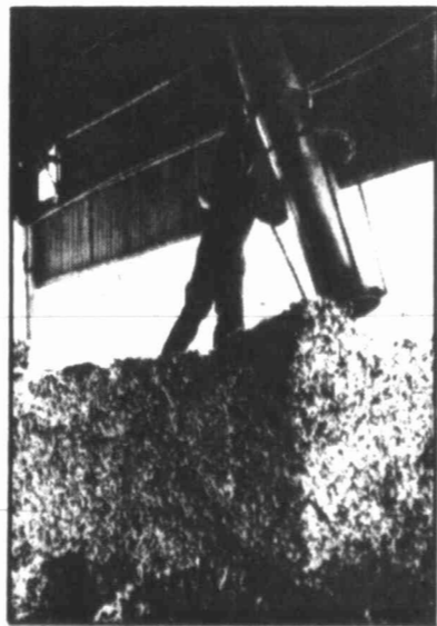
A suction pipe vacuums cotton into the Luther Gin for cleaning and baling.
