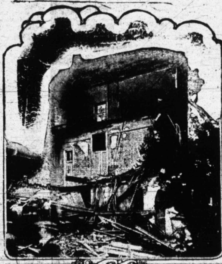
RUINS OF SAUL BUILDING WASHINGTON WHERE SEVERAL WERE KILLED
