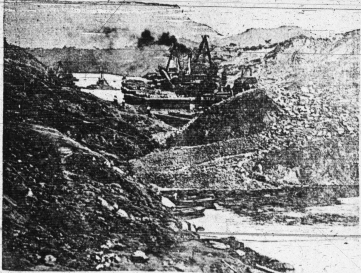
PANAMA CANAL CHANNEL BLOCKED BY SLIDE
