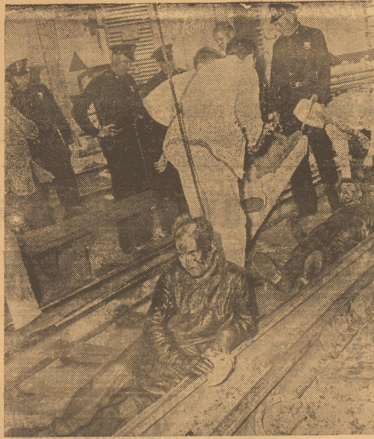
PAINTERS HURLED TO TRACKS . . . Two painters, Harry Paravolos (left) and Frank Pavich, working on the underside of the Melrose Ave. bridge at the New York Central yards, Bronx, N. Y., await removal to Morissania hospital after they were hurled about 25 feet to the tracks when their scaffold slipped. The injured victims were covered with the black paint they were using to paint the bridge. Police stand by as doctors prepare stretchers for their removal to hospital.
