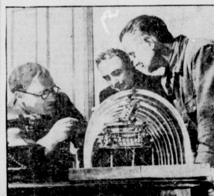
FOR MINE SAFETY—At the New Crosshairs Colliery, British coal miners, the inventors of a power-operated support to guard coal miners from cave-ins resulting from boring or blasting examine a scale-model. Named the Tromit, the steel-arched safety device is operated by remote control.
