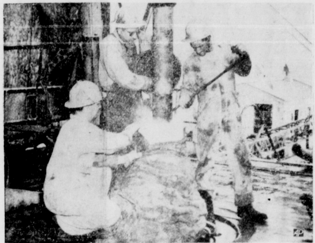
PACKED IN ICE—When normal methods of preventing a threatened blowout of an oil well 7 miles off shore at Grand Isle, La., failed to get results, the drilling crew turned to powdered ice. The ice pack plugged the hole by freezing the mud that had packed into the drill pipe. Success of the operation was credited with preventing possible severe damage to three producing wells on the offshore drilling platform that cost $1,500,000 (m). The ice trick is not new to the oil industry, but it is a procedure that is used only on rare occasions. (AP Photo)
