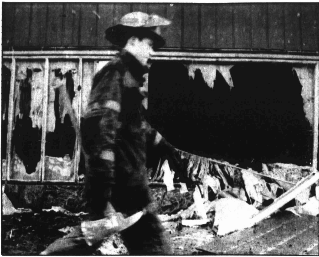
A firefighter with an axe in hand walks by the wreckage of the St. Vincent de Paul Society's clothing outlet and warehouse in Detroit Saturday. About 100 firefighters responded to the five-alarm blaze which cause $1 million in damages. The cause of the blaze is not yet known.
