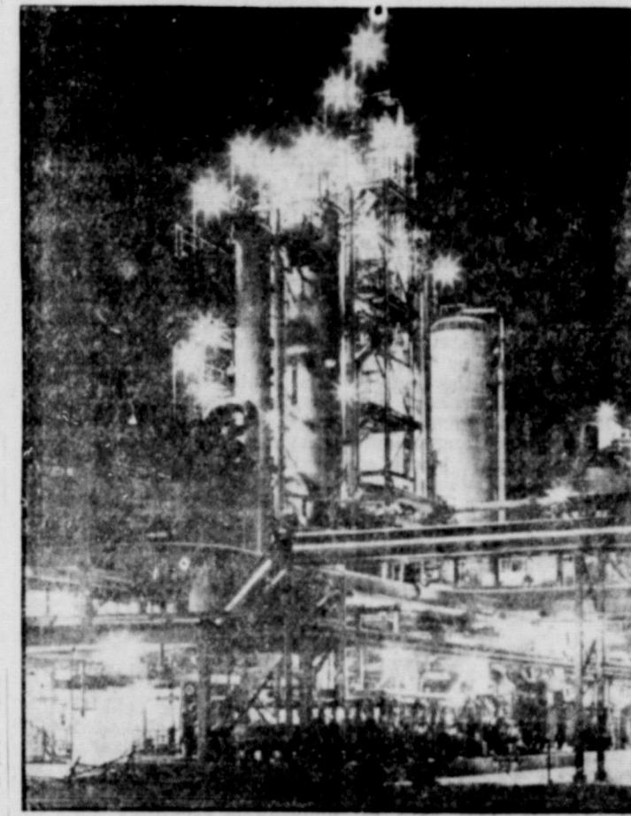
IT'S TEXAS, NOT TIMES-SQUARE — The lights of a new lubricant refinery at Beaumont, Tex., blaze in the night. These bright lamps are in the plant's phenol unit where petroleum is treated to free high-quality oils by dissolving low-quality oil.
