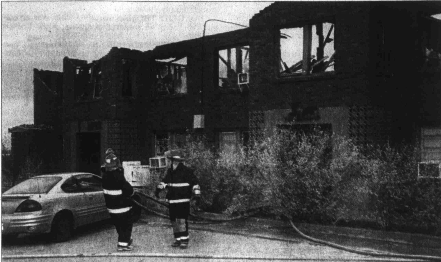
HERALD photo/Thomas Jenkins Firefighters clean up the remains of an apartment complex at the intersection of Eighth Street and Nolan after an early morning fire ripped through the structure.
