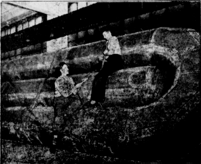
Massive rubberized cotton pontons like the one above aid in giving added mobility and striking power to U. S. armored forces. By the use of such pontons with heavy steel treadways, new armored force bridges can be erected faster and carry heavier loads than any other military bridge in existence.
