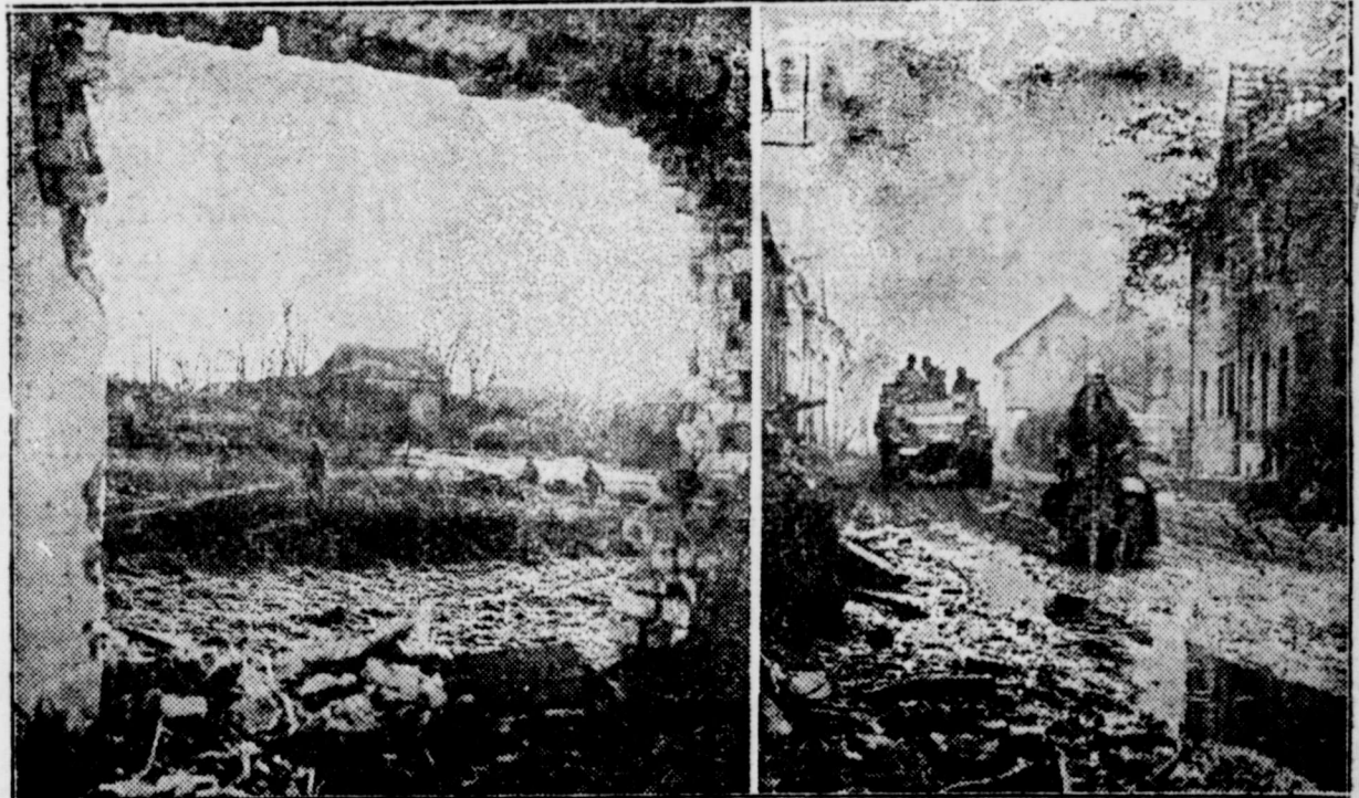
Released by U. S. War Department, Bureau of Public Relations. ONWARD INTO GERMANY—Left, four U. S. Army infantrymen, framed by the shattered walls of a wrecked building, as they file through an open area in Puttrelange, France. Right, Vehicles move through Beggendorf, Germany, as the new offensive inside Germany gets under way.
