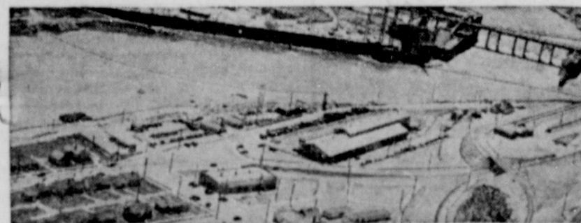
It's only a step from Grand Coulee homes to the dam site.
