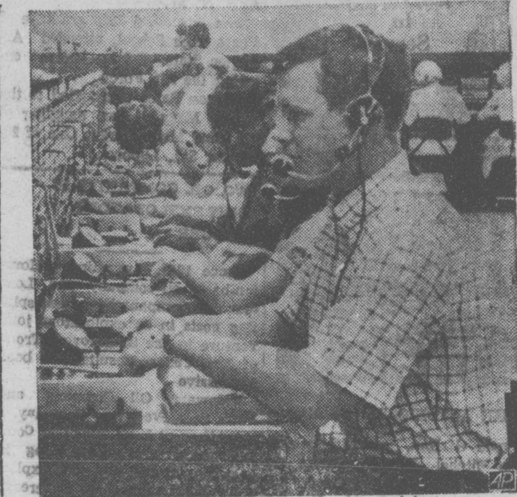
AGGIE BREAKS TRADITION — Don Kilfoyle, Texas A&M University junior electrical engineering major, is shown at his post on the switchboard at Southwestern State Telephone Co., Bryan office. Kilfoyle invaded the all-female field after applying for a part-time job with the company to do something in electronics. (AP Wirephoto).
