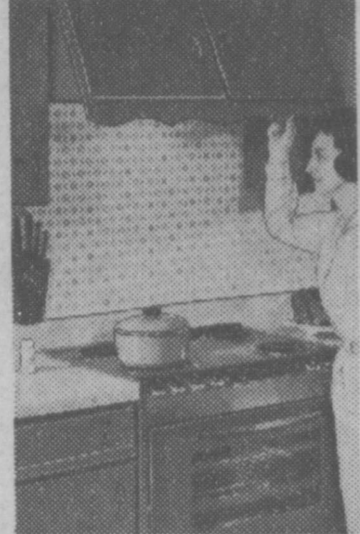
CABINET FRONT converts to a modern range hood with a slight pull forward, giving ventilation and complementing kitchen built-ins. "Kenmore Hide-A-Hood" at Sears.
