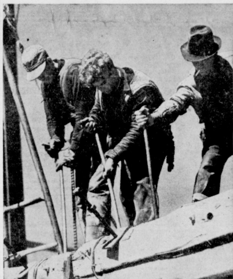
Work has just started on a new contract to place 6,000,000 cubic yards of concrete in the dam and west powerhouse, increasing the height to 553 feet. Successors to the beaver are the form raisers (above) who shift forms
